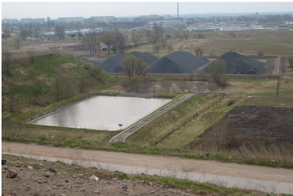
Fig. 4. The tank for leachates from the old landfill (zone RL – site VI) (phot. A. Kalwasińska)
