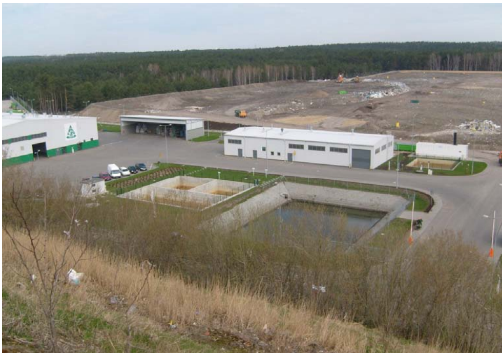
Fig. 2. The new, operative landfill (zone NL – sites I, II and III) (phot. A. Kalwasińska)
